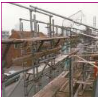
Figure 16. A hoist-console scaffolding
