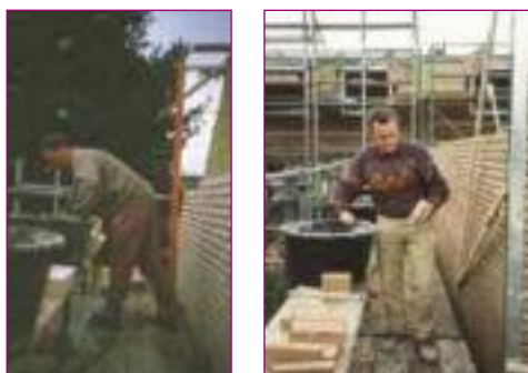
Figure 15. Raised bricklaying
